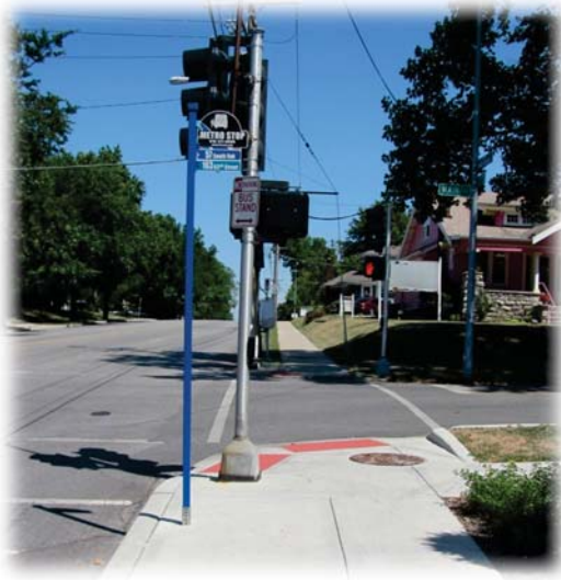
Figure 3-5: Example of intersection issues
