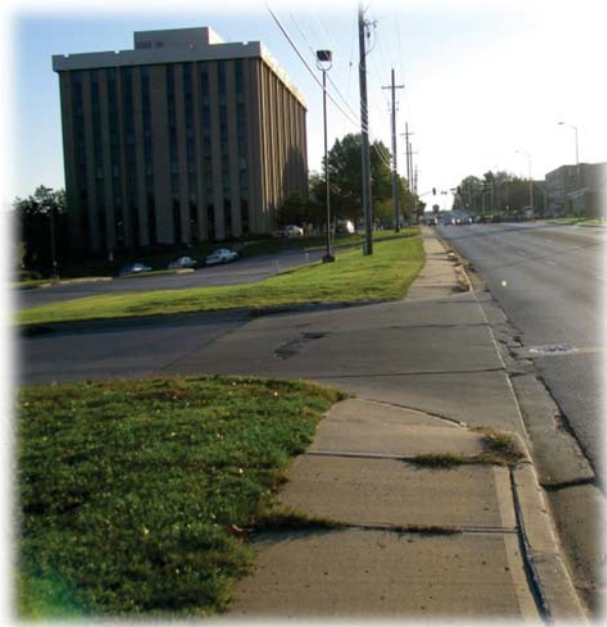
Figure 3-4: Example of sidewalk issues
