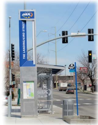
Figure 2-5: KCATA MAX Troost Line facilities
