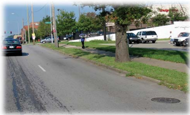
Figure 3-2: Example of curb issues
