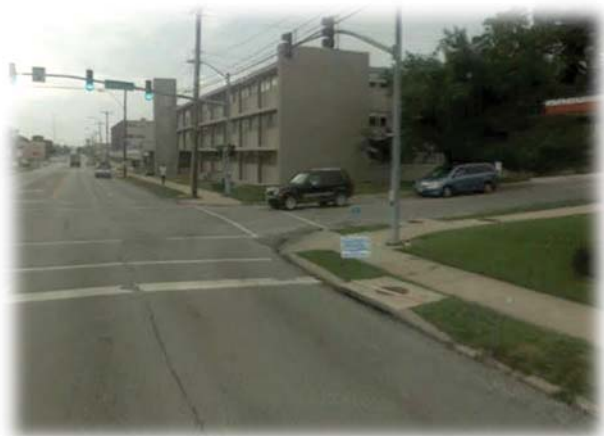
Figure 3-3: Example of storm water inlet issues
