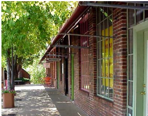
Awnings and canopies should be integrated in buildings along facades that front pedestrian walks.
