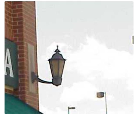
Façade-mounted lighting enhanced the illumination level along the block face.
