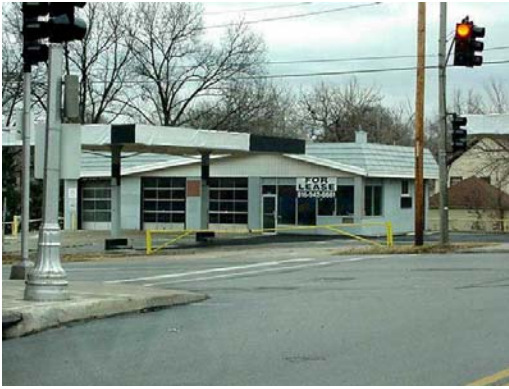
Some properties in the envisioned Oak Street Neighborhood Village afford opportunities for redevelopment.
